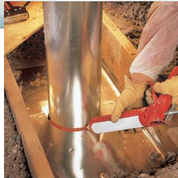
Seal with metal collar, high temp. caulk. Add metal insulation dam
