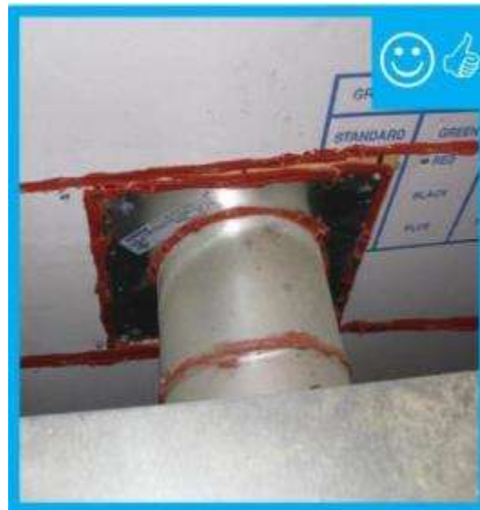
Big square hole around round chimney
