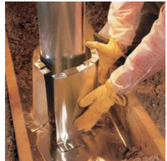
Seal with metal collar, high temp. caulk. Add metal insulation dam
